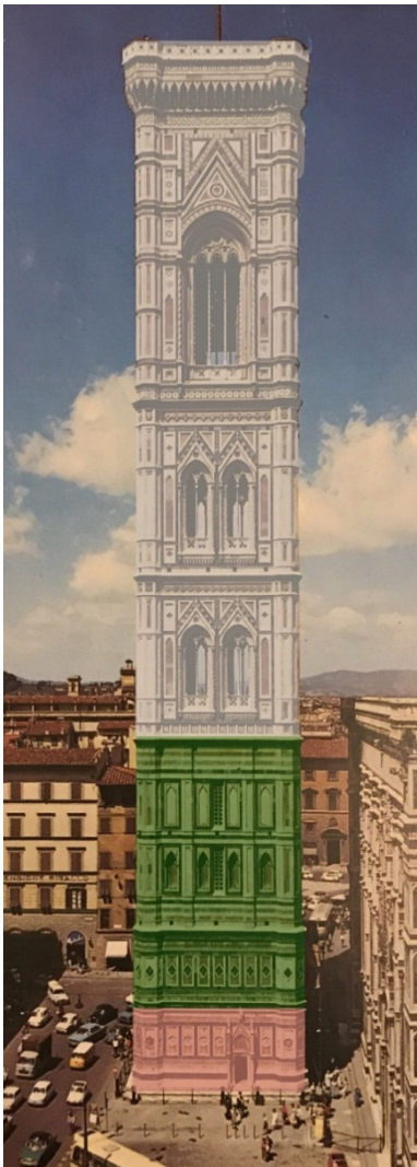
Figure 1- The Giotto Bell Tower in the downtown Florence; different colours are used to highlight the different construction phases: Giotto 1334-1337 phase in pink; II phase by Andrea Pisano 1337-1343 in green, III phase by Francesco Talenti 1343 - 1359 in gray.
