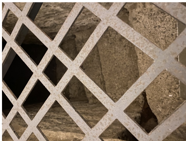
Figure 9. Lecce Cathedral: photo related to the chamber evidenced by GPR surveys.
