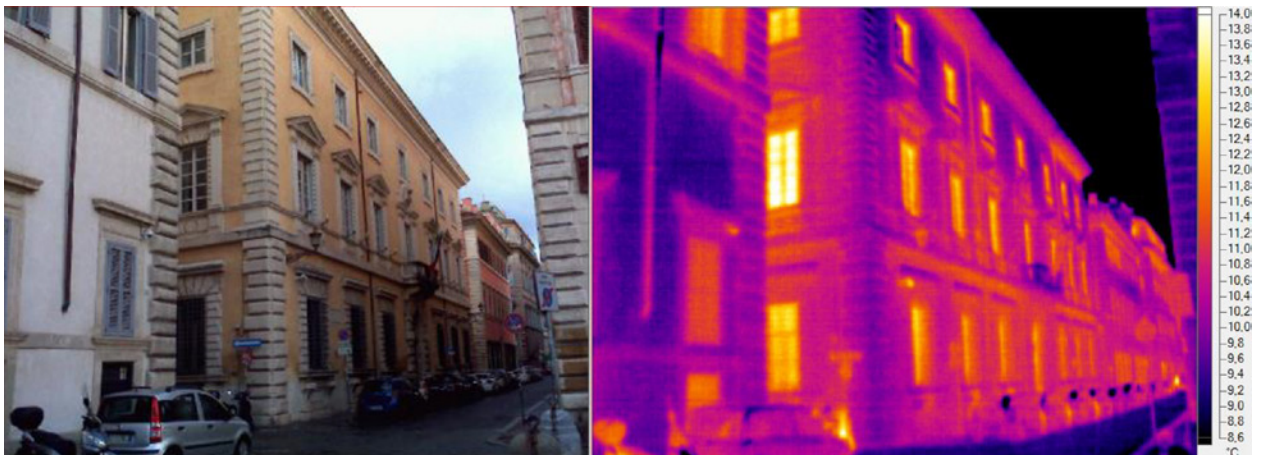
Fig. 6. Comparison between the photography and the termographic image of the main façade of Palazzo Maffei-Borghese, Rome
